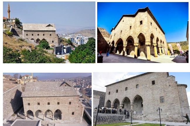
Figure 15. Photo of the church after restoration [29, 35, 36].
