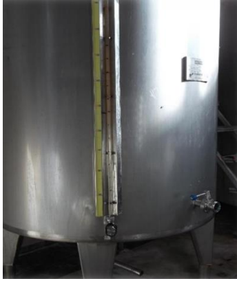
Figure 3. Clarification and deacidification tank [6]
