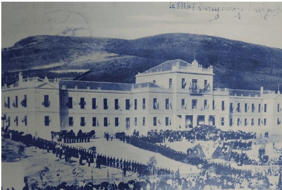
Image 1. Hospital general, front facade (Michaleas and others, 2022, p. 3)
