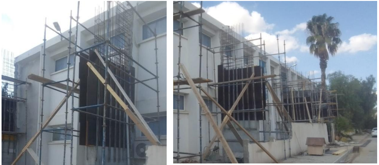
Figure 7. Shear wall added to classroom, a) Block B, b) Block A
