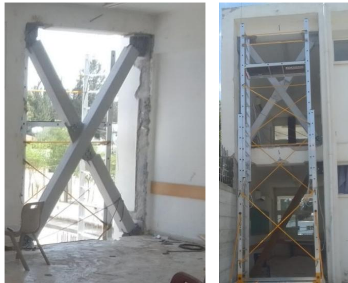
Figure 8. Tube 200x200x12.5 X-braced frames added to classroom, a) Block A, b) Block B
