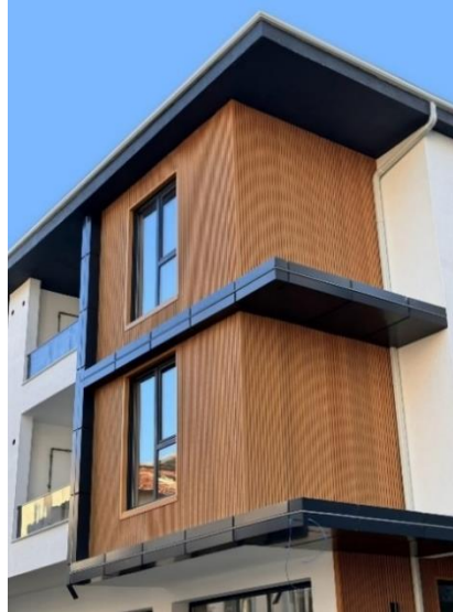
Figure 5. Application of wood-plastic composite as an exterior building cladding (URL-15, 2024).
