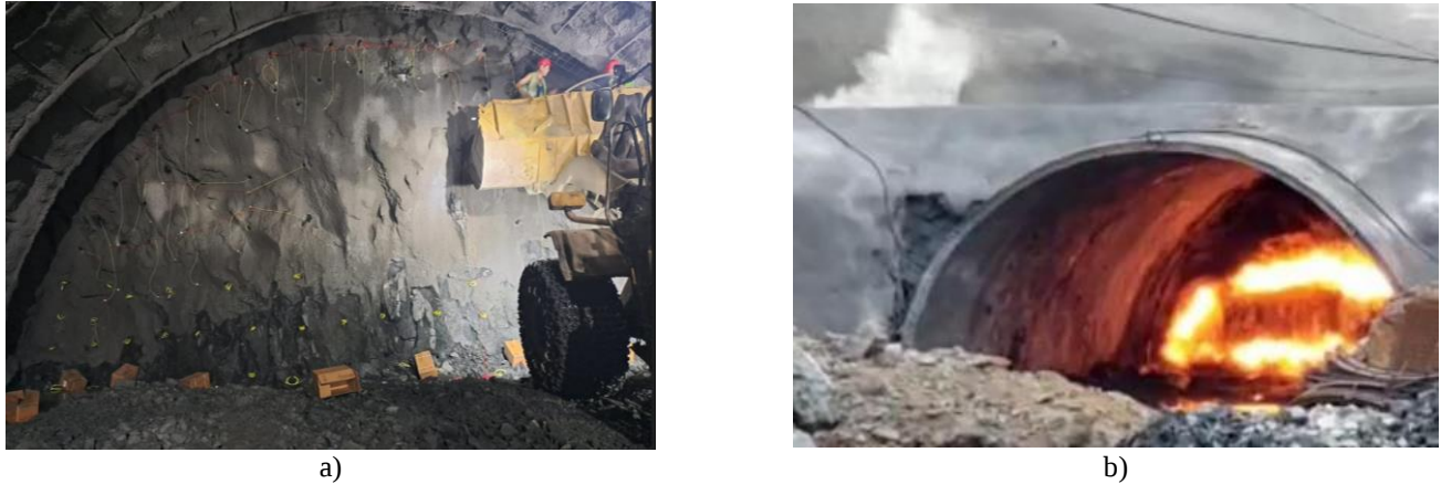
Figure 20. (a) Blasting material placement (b) Blasting
