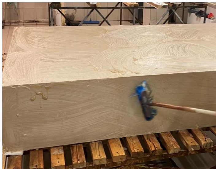
Figure 9. Brushing the GFRP panel surface with the chemical solution
