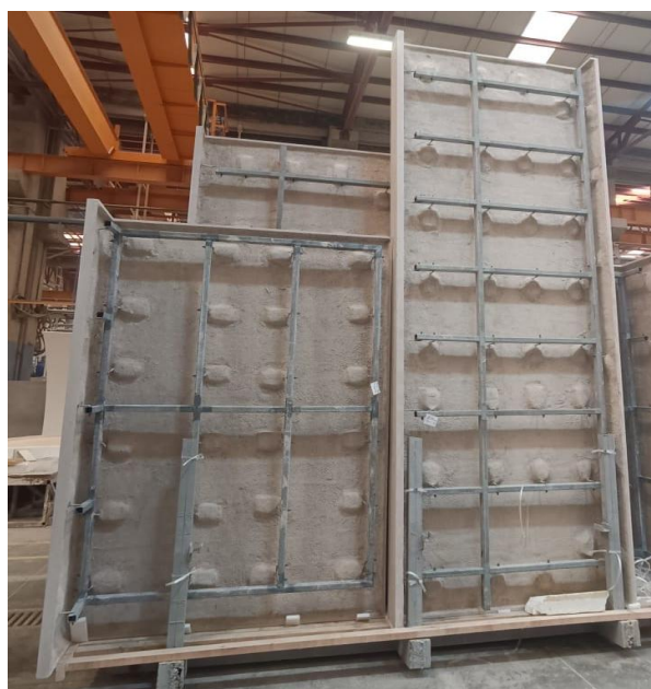
Figure 4. Metal anchors behind the GFRC panel
