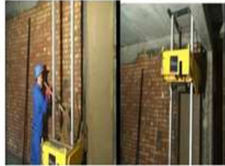
Fig. 5. Wall Plating with Machine Aid
