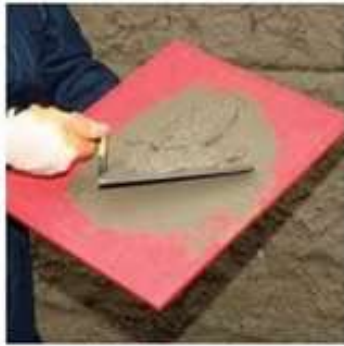
Fig. 4. Wall plastering using trowel
