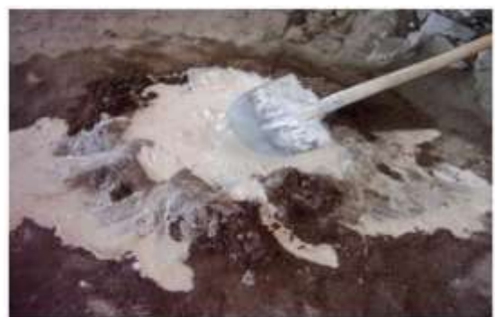
Fig. 7. Mixing of sand and lime
