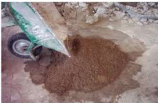
Fig. 6. Preparation of sand for fine plaster mortar
