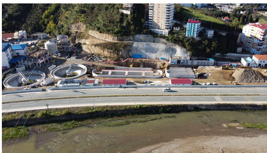
Figure 1. The general view of the Giresun WWTP
