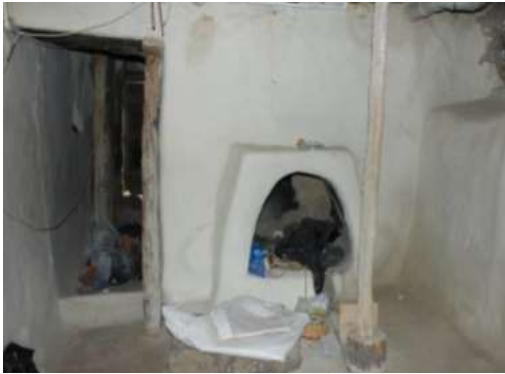
Foto 3f. Zemin kat oda ve kerpiç ocak (Photo 3f. Ground floor room and adobe stove)
