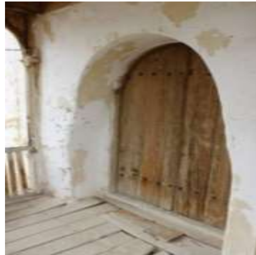
1s. Gezemek/balkon girişi (Photo 1s. Balcony entry)
