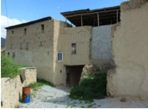
Foto 3d. Kuzeybatı cephe (Photo 3d. Northwest front)
