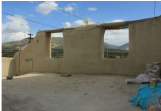
Foto 3n. Birinci kat hayat (Photo 3n. First floor living)
