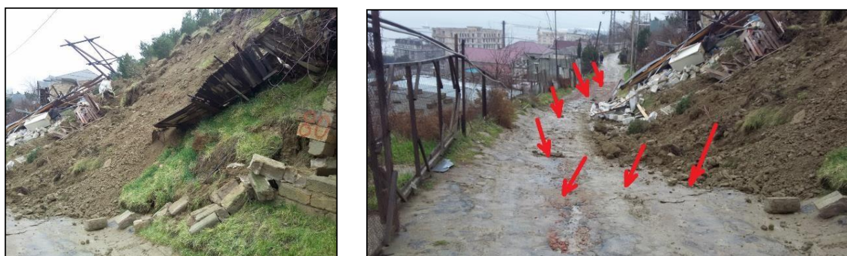
Fig. 17. Destruction, observed cracks and uplifts on the surface at a distance of 130 m from the edge of the landslide
