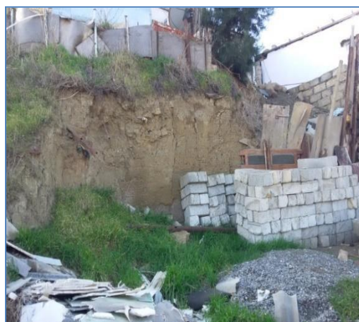
Fig. 7. Slope cut in front of the landslide zone
