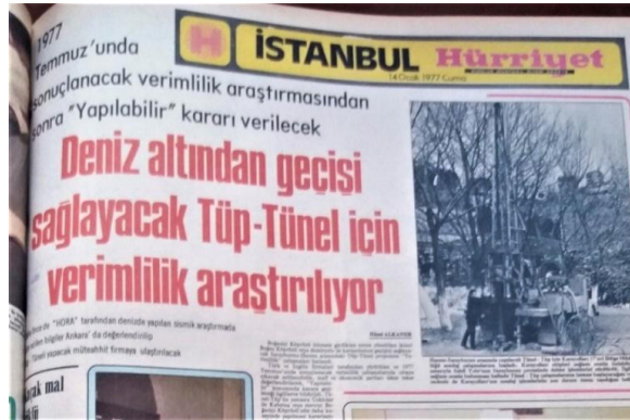
Picture 7. Construction of a tube passage in the Bosphorus (Hürriyet, 14 January 1977).
