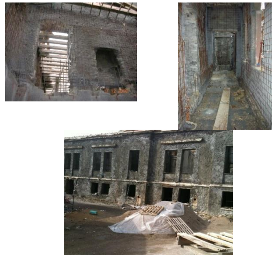
Figure 6. RC jacket applications in listed stone masonry buildings in Greece
