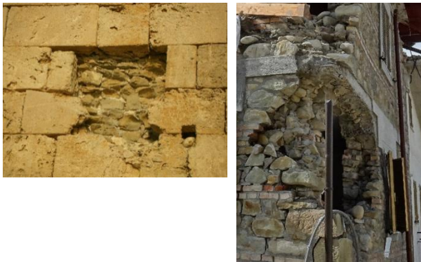
Figure 2. Delamination of three-leaf masonry and damage due to seismic actions in Amatrice and in Samos
