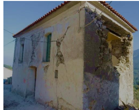
Figure 2. Delamination of three-leaf masonry and damage due to seismic actions in Amatrice and in Samos
