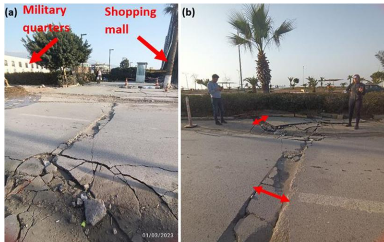
Figure 2. Liquefaction-linked damages observed around the Iskenderun Bay during the first main Kahramanmaraş earthquake event
