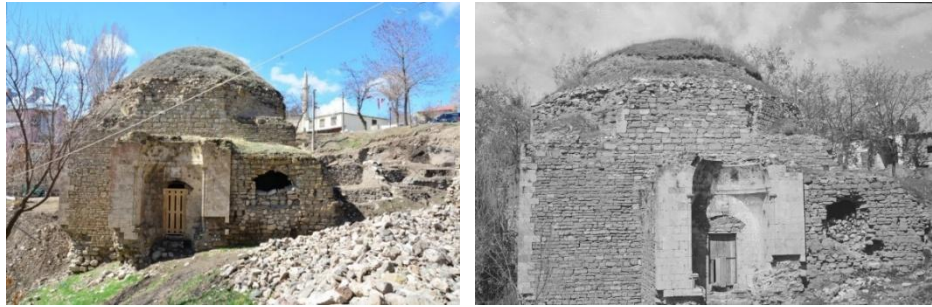
Figure 6. General views of the main gate from the east
