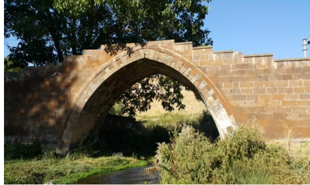
Figure 1. Emir Bayındır Bridge
