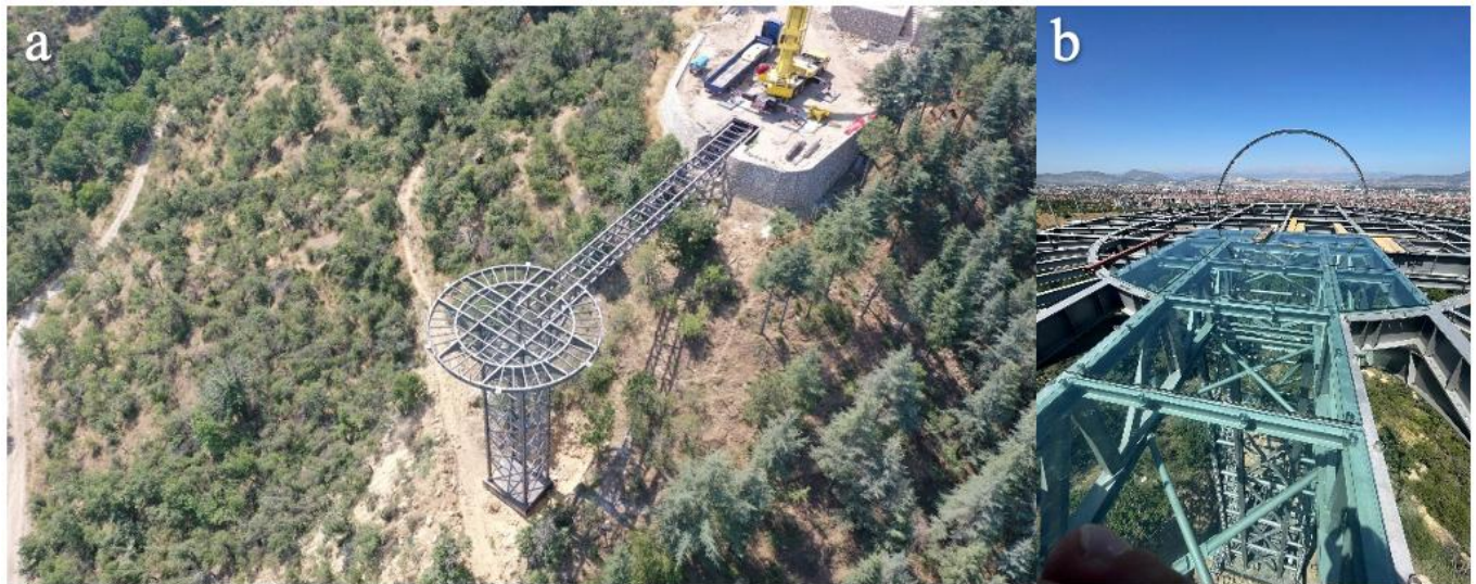
Figure 3. a. Construction Process of the Steel Support Frame of the Glass Platform, b. Assembly Phase of the Completed Walking Axis and Glass Surfaces (Isparta Municipality, Directorate of Survey and Project, 2023)
