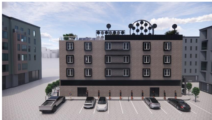
Figure 5. Overall view of a building with renewable energy generation for EV charging.
