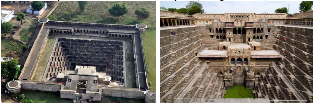
Figure 2. Stepped water well in Rajasthan, India [URL2]
