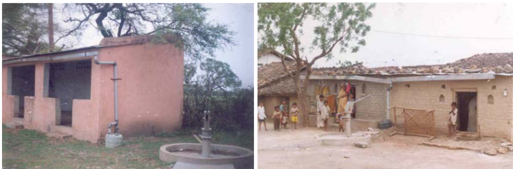
Figure 1. Rooftop water collection technique used in Madhya Pradesh villages ( Technical Document, 2004 )
