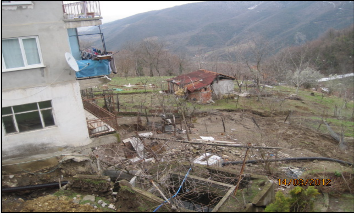
Şekil 5. Hamidiye köyünde meydana gelen heyelan Figure 5. Landslide occurred in Hamidiye village
