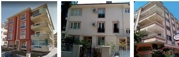
Figure 5 Apparent Quality Evaluation (a, b, c) and Short Column Effect (c) Examples
