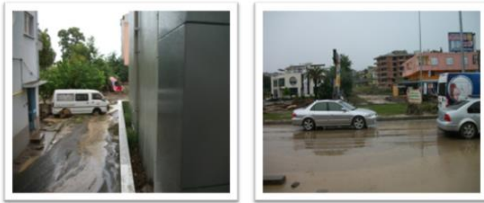
Figure 14. The Damages Caused by the Flood of Degirmen Stream
