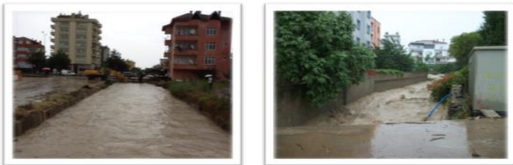
Figure 13. The Damages Caused by the Afanlı Stream Flood
