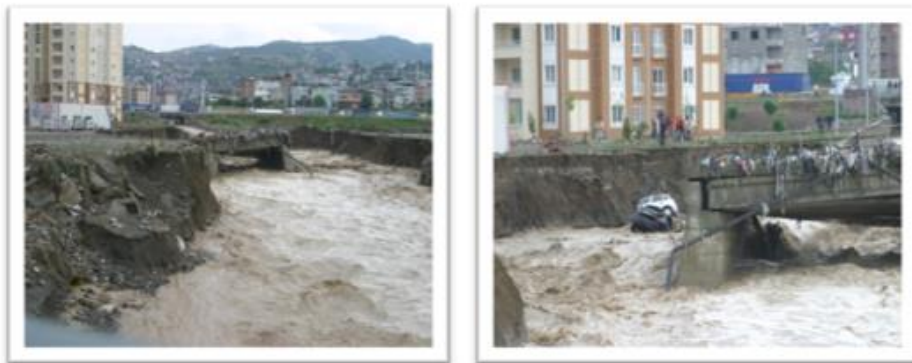
Figure 10. Damages of Yilanli Stream Flood in Canik District
