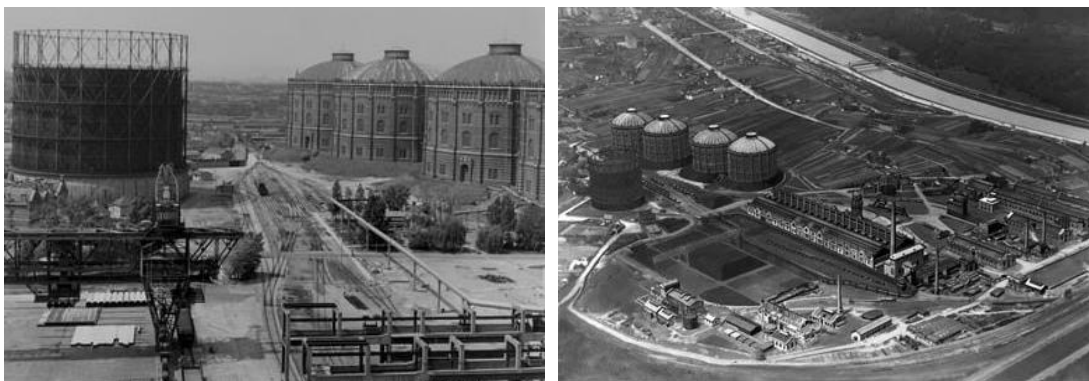
Figure 19. Four gasometers were built in a period of three years, between 1896 and 1899 [36]
