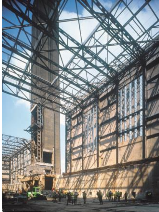
Figure 13. Steel frame, central chimney and brick facade construction [32]
