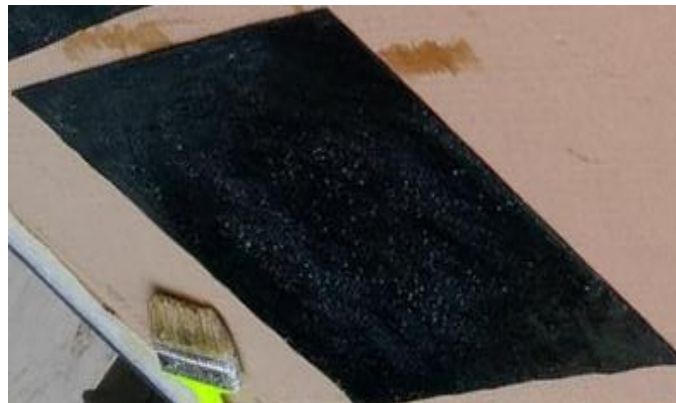
Figure 4. Application of adhesive onto the waterproof membrane
