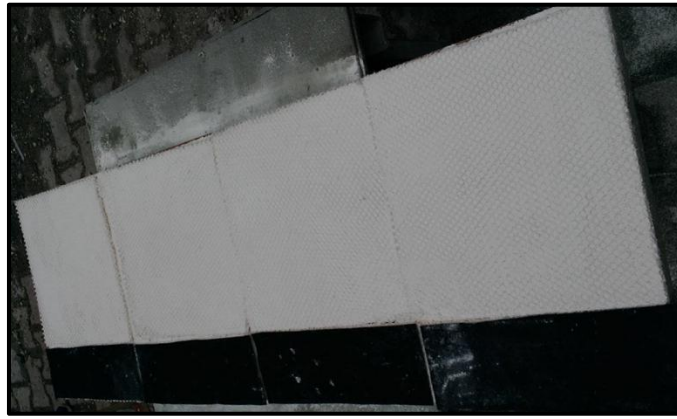
Figure 5. Adhesion of the waterproof membrane onto the surface of the 3D textile
