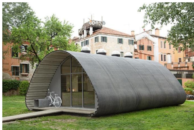
Figure 2. Example of tiny houses constructed with 3D textile concrete [15].
