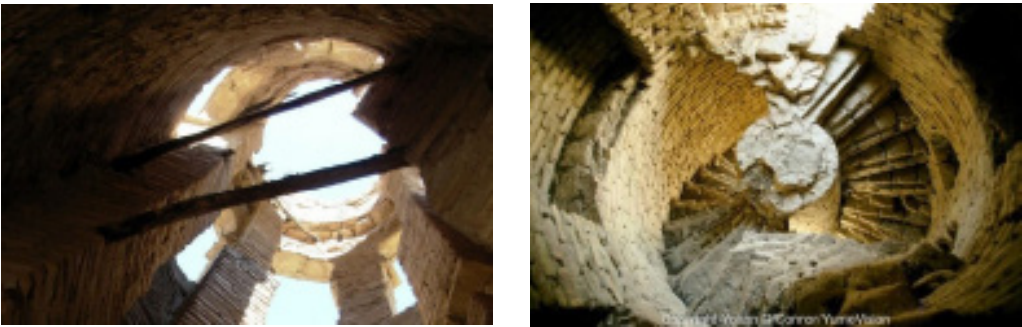
Figure 7. View of the Jam Minaret's upper body (petek), staircase, and core (wikimedia.org; photoshelter.com).
