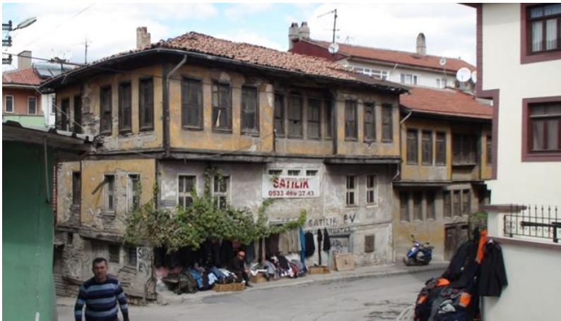
Figure 8. Old Turkish house between irregular new buildings in one of center neighbourhood, source; author
