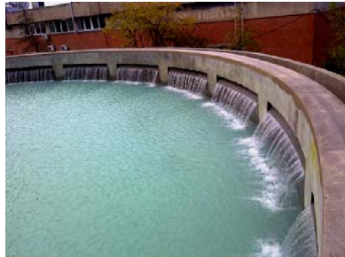
Figure 9. Water treatment facilities after repairing (Kabashi at.al, 2014)
