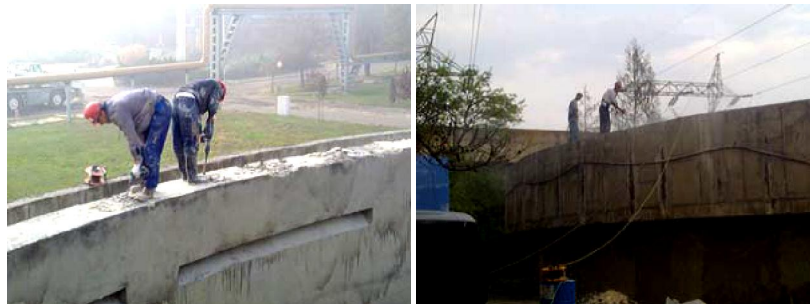
Figure 7. Removal of the damaged parts and the cleaned concrete surface inside.
