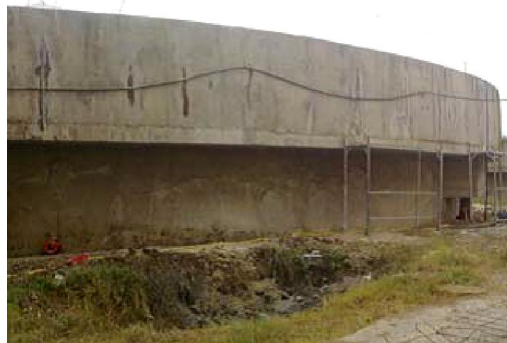
Figure 6. The concrete structure during the visual inspection: outside and inside.
