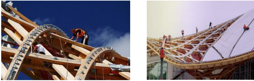
Figure 11. Wooden frame and roof system (URL11)
