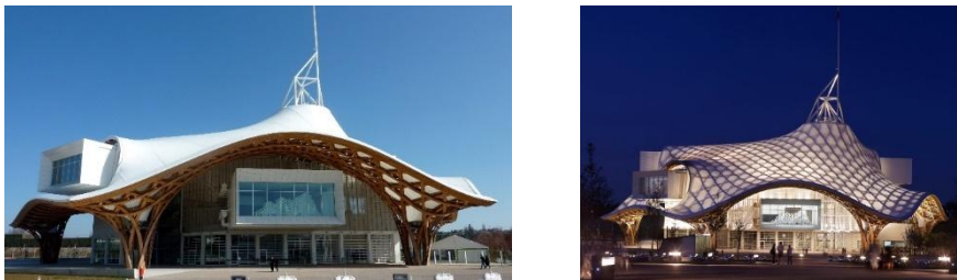
Figure 9. The Centre Pompidou Metz (URL9)
