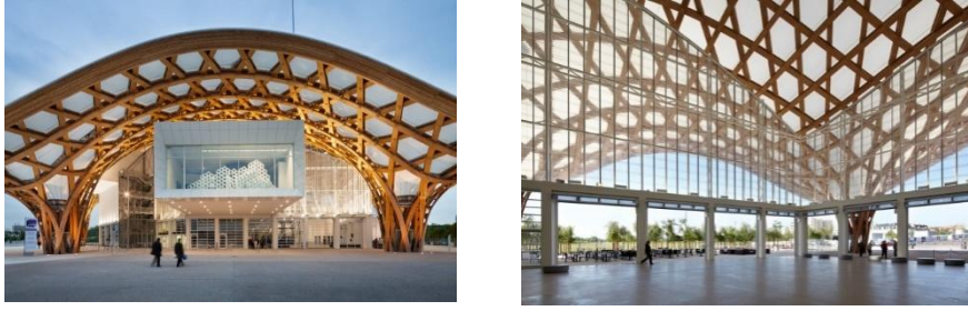
Figure 13. The Centre Pompidou Metz's main entrance and hexagonal wooden braiding in its interior (URL9)
