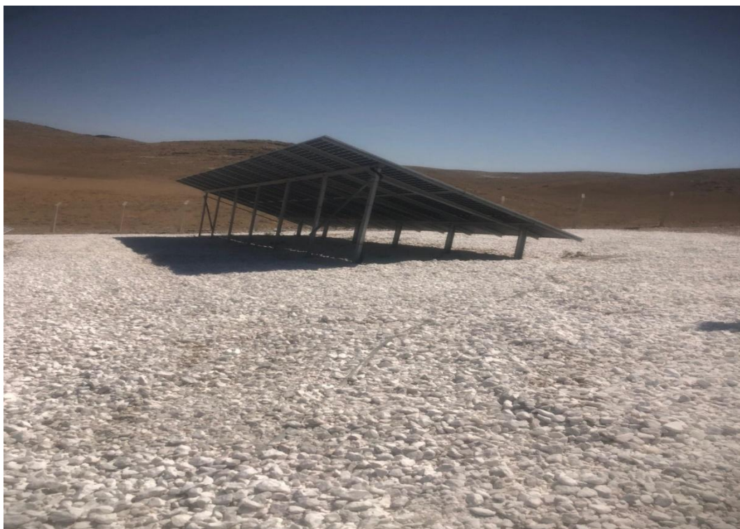
Figure 1. Application of high-reflectivity white gravel (albedo \approx 0.50 ) beneath bifacial PV modules
