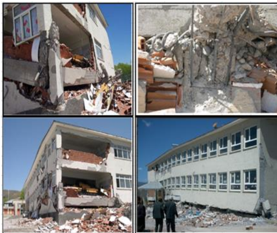
Figure 1.Çeltiksuyu Regional Primary Education School Building
