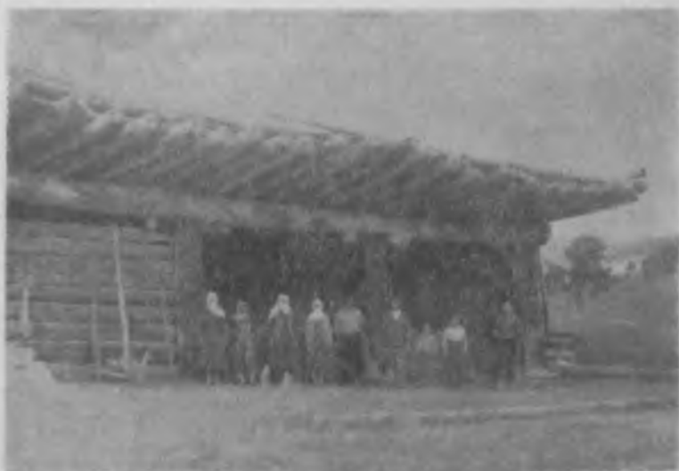
Photo 10. A wooden dwelling (house) in the Mekpur mezraa, at an altitude of 2000 m, 9 km north of Lake Tortum. The house has two sections, one of which belongs to animals to/for shelter or refuge and the other section belongs to family of peasant (at right).
