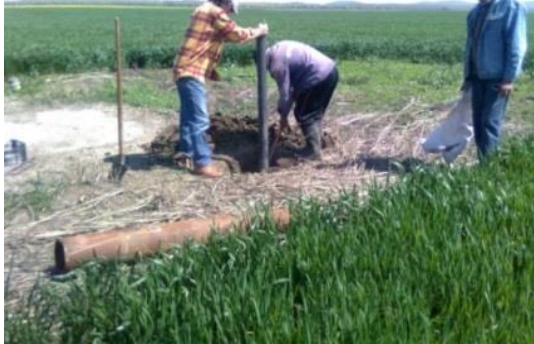
Figure 7. Photo documents – Assembling of hydrogeological well
