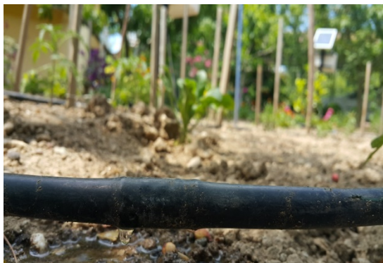
Figure 8. The view of the drip irrigation system
