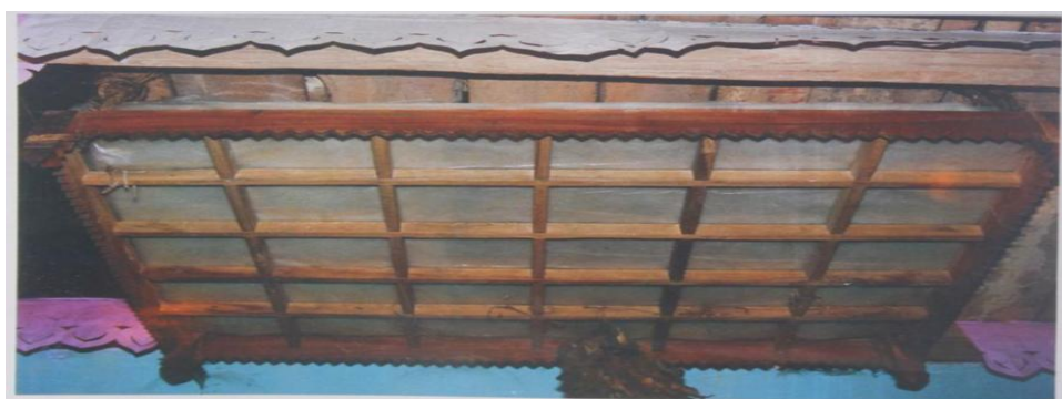
Figure 2. Traditional wooden Matoli frame
