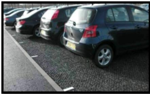
Figure 2: Permeable gravel filled parking lot of Bristol & Bath Science Park in conformance with the principles of SuDS for 200 cars (Gravel-filled porous car parking, 2016)
