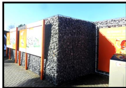
Figure 14: Examples of gabion walls which we recently see often in our day, Den Haag (Photo: Şentürk, 2015)
