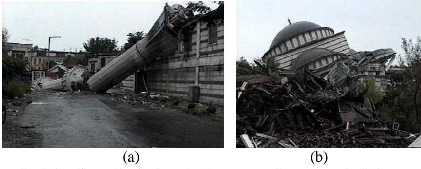
Şekil 2. Minare devrilmiş ve kırılmış ve cami yan yatarak yıkılmış. Figure 2. The minaret is overturned and broken and the mosque is lying down on its side
