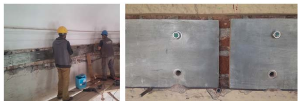
Picture 15 – Reinforcement (Stainless Steel) Manufacturing
