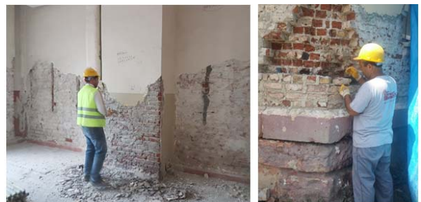
Picture 14 -Wall Masonry
