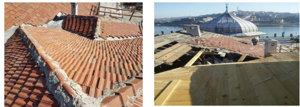
Picture 11 - Roof Dismantling Production
