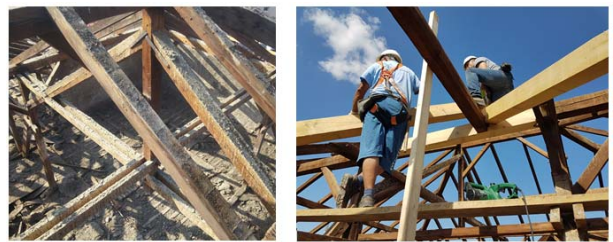
Picture 12 - Replacement of Roof Materials
