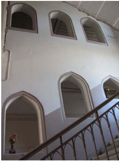
Figure 8 – Openings in the main staircase wall
