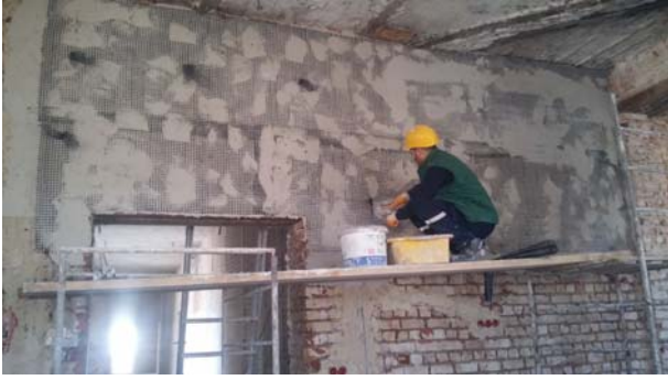
Picture 16 – Reinforcement with Carbon-fiber Network
