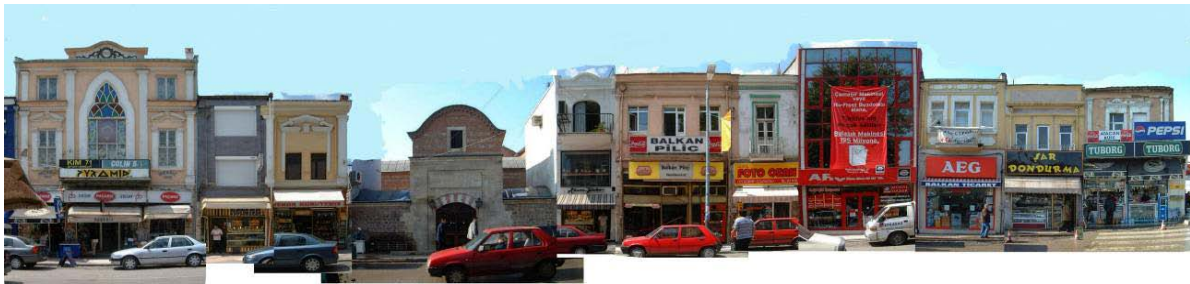
Figure 10. Heavy motor vehicle traffic along Saraçlar Street
