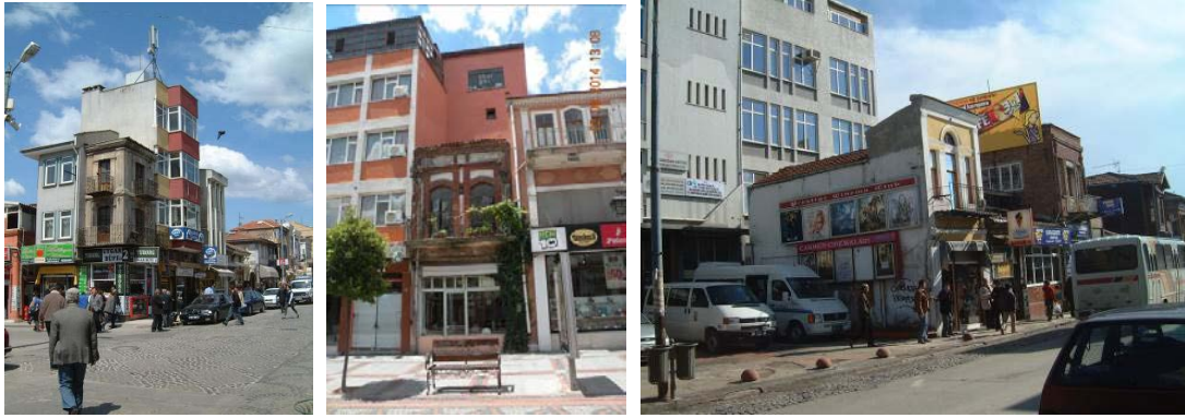
Figure 6. Examples of building height violations along Saraçlar Street.
