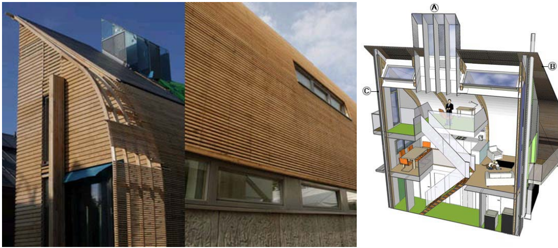
Figure 15. left: first zero-emission, eco-friendly office; right: First zero-emission, eco-friendly office A. Wind catcher; ventilation means in summer season. B. Solar collectors, hot water and power generation means. C. High amounts of heat insulation [18].
