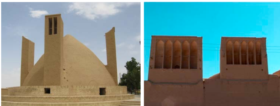
Figure 3. View of wind catcher type 1: one sided; right picture: A view of a one-sided wind tower in Ardakan city, Yazd province, Iran [7]
