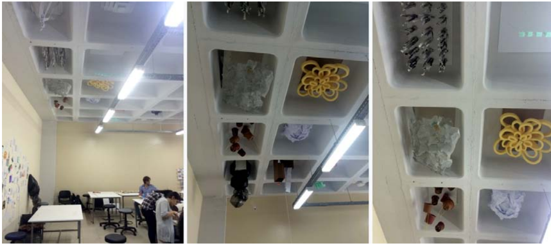
Figure 8. On-site infill installation to the void, group work
