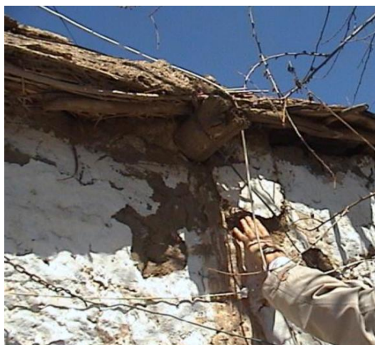
Figure 9. Sampling from the South Facade
