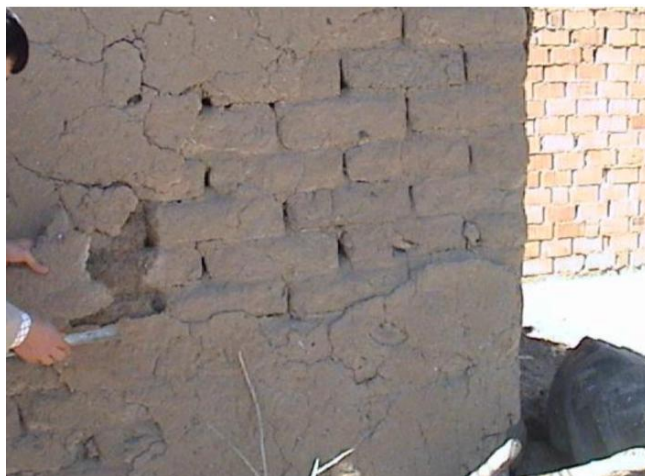
Figure 8. Sampling from the South Facade
