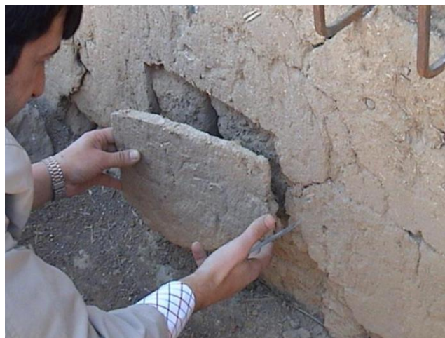
Figure 7. Sampling from the North Facade
