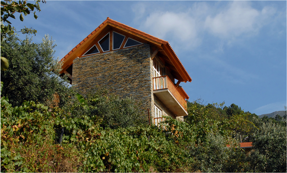
Figure 13 Expansion of the house: local materials and technological innovation. Source: Author's Personal Achieve
