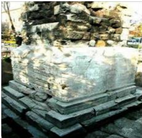
Figure 3. The “Örme Dikilitaş” base component undertook the role of “natural seismic isolator” to dissipate the actions of earthquakes during 1000 years. The previous status of surface of the 1.24 m level of the massive slip stone is not entirely visible.
