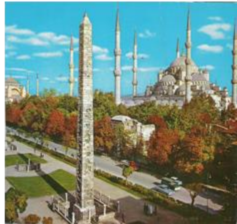
Figure 3. The “Örme Dikilitaş” base component undertook the role of “natural seismic isolator” to dissipate the actions of earthquakes during 1000 years. The previous status of surface of the 1.24 m level of the massive slip stone is not entirely visible.
