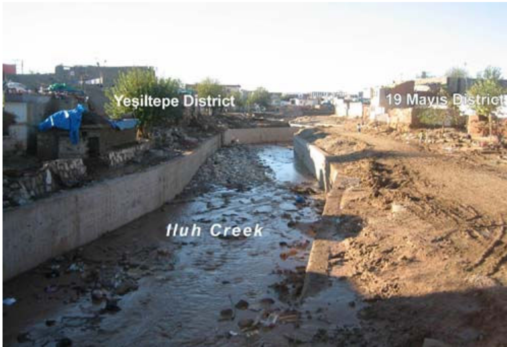
Figure 16. Canal of Iluh Creek flowing through city center of Batman that filled up with flood debris in the flood event on October 31-November 1, 2006.
