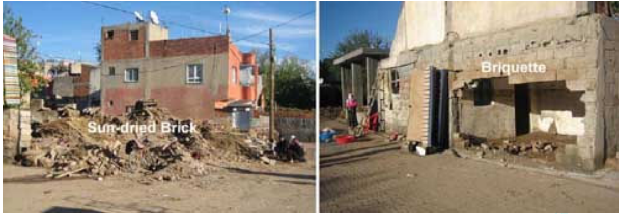
Figure 9. Dwellings made of adobe brick and briquette on the stream bed of Iluh Creek that were affected by the flood in Batman in 2006.
