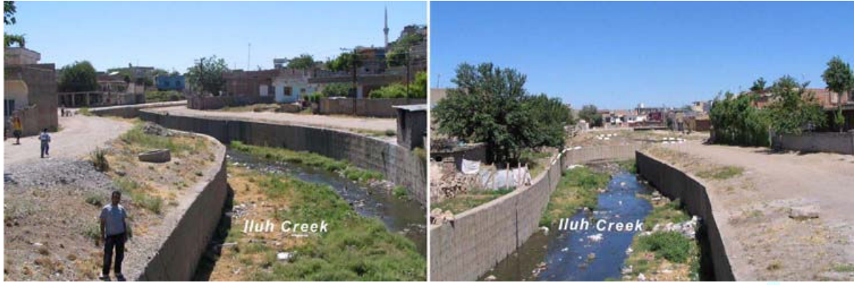
Figure 15. Sinuous structures on the canal of Iluh Creek between the districts of 19 Mayıs and Yeşiltepe.
