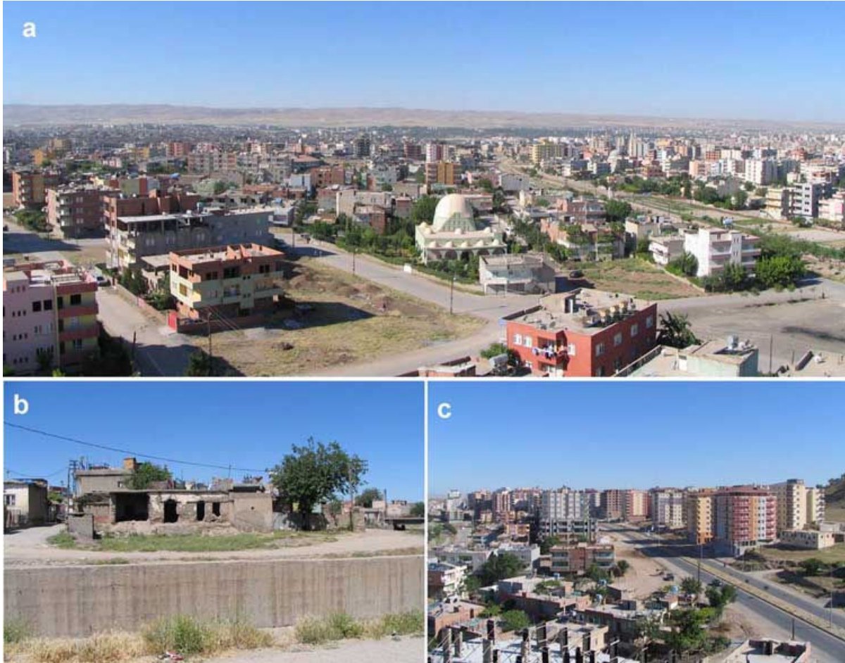
Figure 8: Dwelling types in different districts of the city center of Batman. a) Multi-storey buildings constructed in the north of the city in recent years and single-storey dwellings in the south. b) Dwellings constructed illegally and severely damaged in the flood disaster of 2006. c) Modern buildings constructed in the northern part of the city in recent years.
