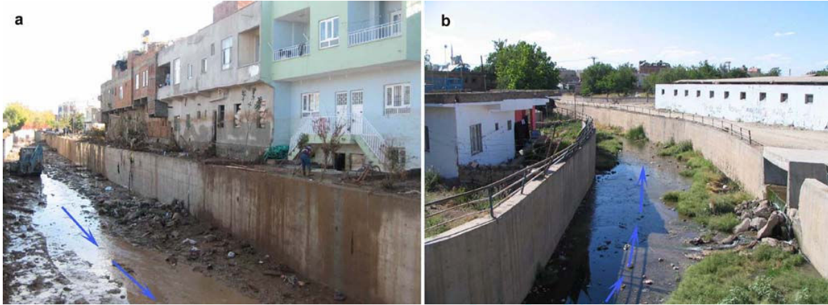
Figure 10. Settlements constructed on the flood bed of Iluh Creek affected by the flood event in 2006. a) Dwellings constructed adjacent to the canal in the district of Karşıyaka. b) Dwellings restored and re-occupied after the flood event.
