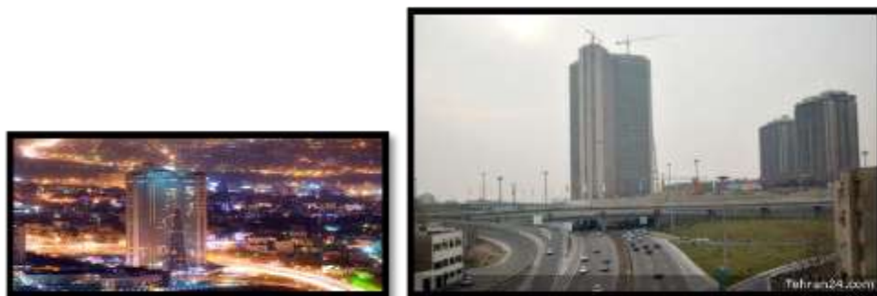
Figure 17. International Tower in Tehran http://wikimapia.org .
