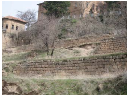
Figure 15. The Levels of the Construction site (Parlak Bıçer, Z. Ö., 2013)
