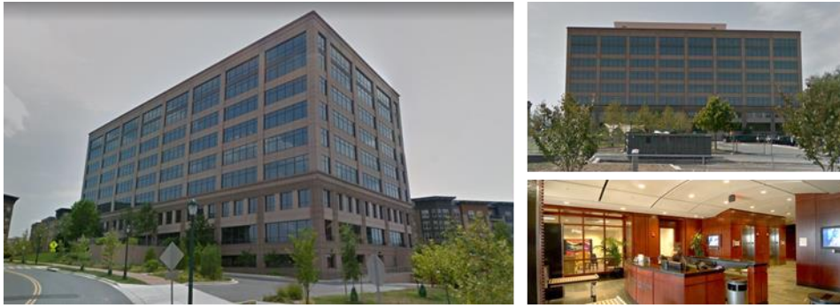
Figure 6. Rockville Office Building [56]
