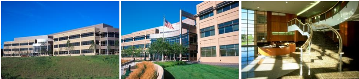
Figure 3. Department of Transportation Lakewood Building [47]
