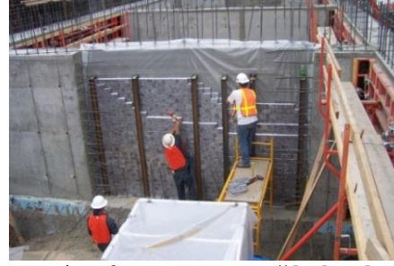
Resim 6. Kurşun tuğlalarla zırhlama [80] (Photo 6. Armoring with lead bricks [80])
