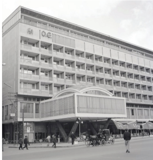
F.13. Scenes showing the V columns in the entrance block and the façade of Eskişehir Porsuk Hotel, 1958 (SALT Research, Gültekin Çizgen Archive)
