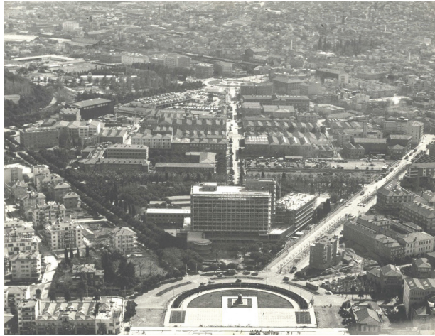
F.15. The Grand Efes Hotel's construction (Kenan Kurtkaya Archive)
