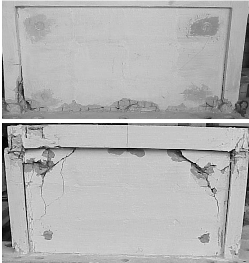
Fig.9. Photographs of first storey infills (CI Specimens)
